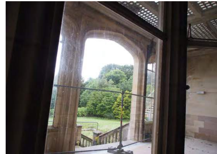
Covered west access from the Ballroom
